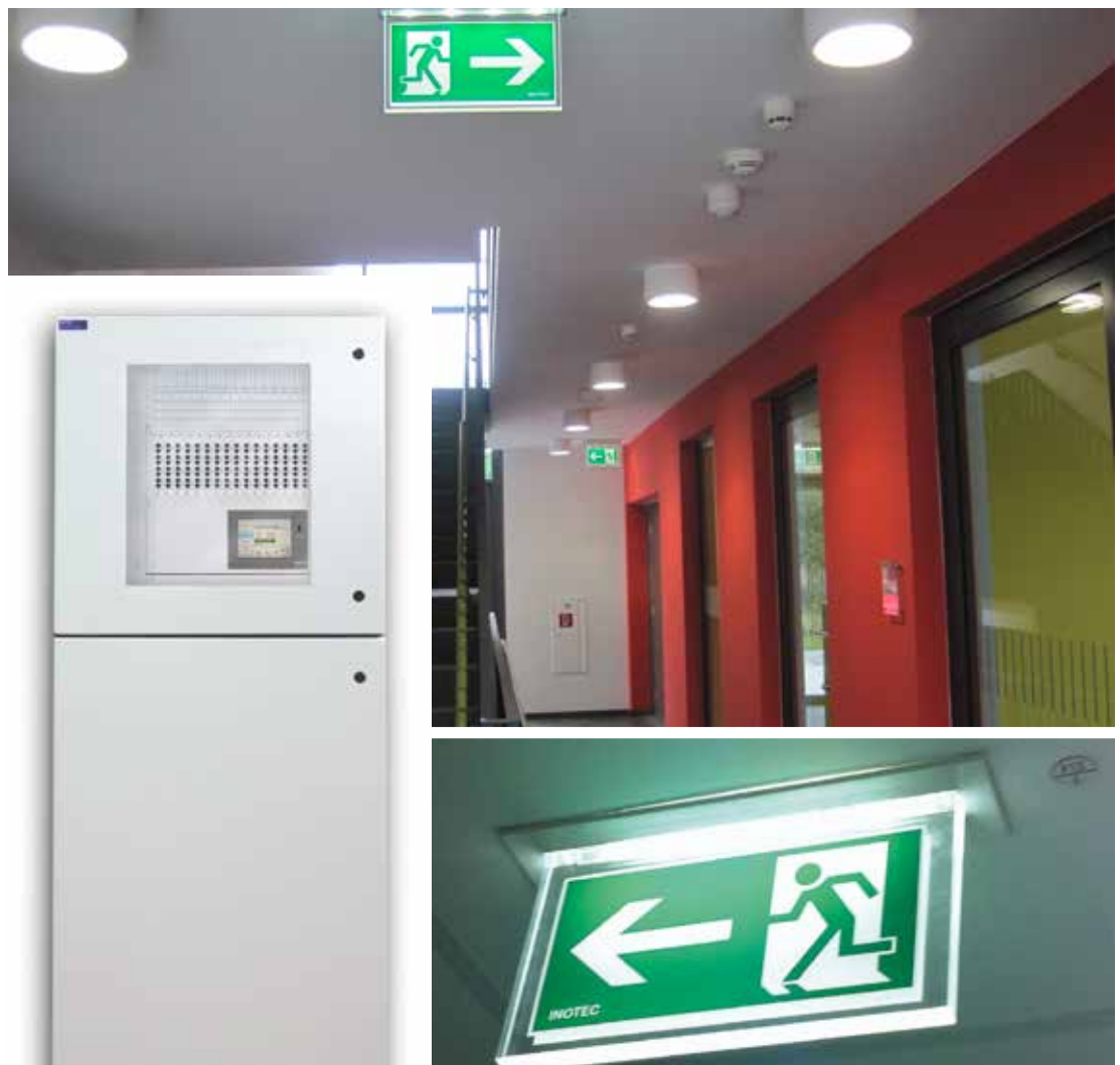
Figure 2: In emergency illumination systems (in the background you see a corridor in the Landesgymnasium für Musik Dresden (Dresden-based music high school of the state of Saxony); the technology was supplied by Klett Ingenieur GmbH) systems of high-capacity common batteries are applied; on the left side you see Inotec's CPS220/64. When, in the case of a mains failure, these batteries have to stand in by supplying emergency power, the fuses may have to be able to cope with high DC short-circuits
